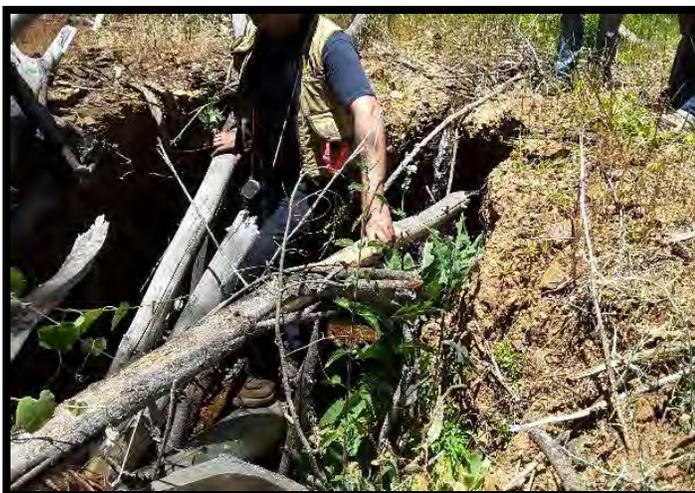
Figure 55. A failed crossing in a post-fire Emergency Notice in the Coast area, where 1-5 yd<sup>3</sup> of sediment were estimated to have been discharged.
