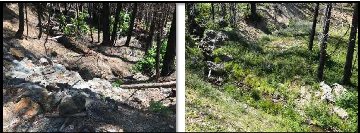
*Figure 54. Armored crossing drainage on a Class III in the Cascade area, left, in a post fire Emergency Notice, that was recorded as having a trace amount of sediment discharge. An abandoned crossing on a Class II post-fire Emergency in the Cascade Region, right, that resulted in less than one yd<sup>3</sup> of sediment discharge based on field observations*
