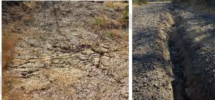
Figure 6: Rills on a road surface (left) and a gully formed on a road surface (right)
