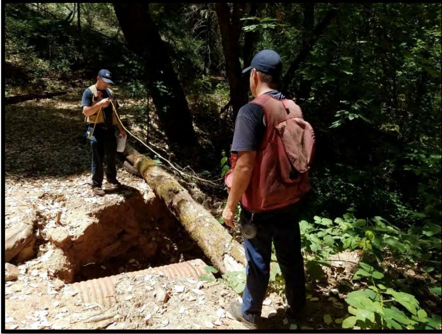
*Figure 53. Overtopped culvert delivering >10 cubic yards of sediment to a Class II watercourse in the Sierra area*
