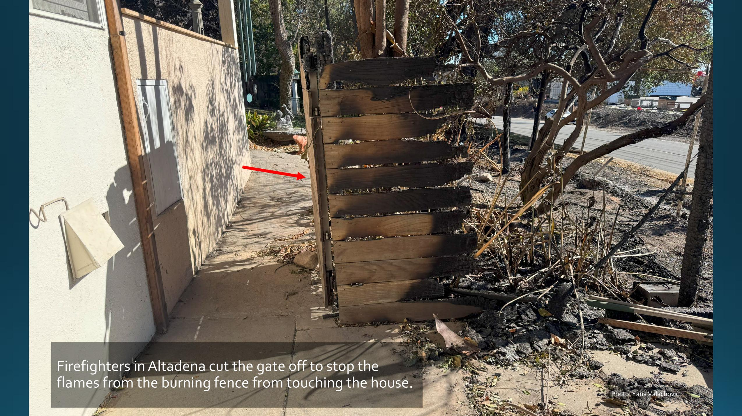
Firefighters in Altadena cut the gate off to stop the flames from the burning fence from touching the house.
