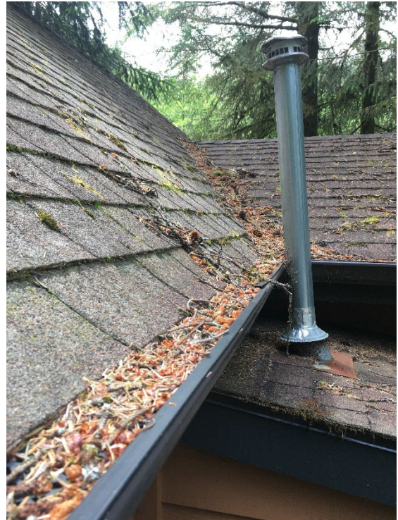
Figure 20. Roof and visible tree debris. Protecting the roof and keeping it clean of debris is an important fire protection action.
