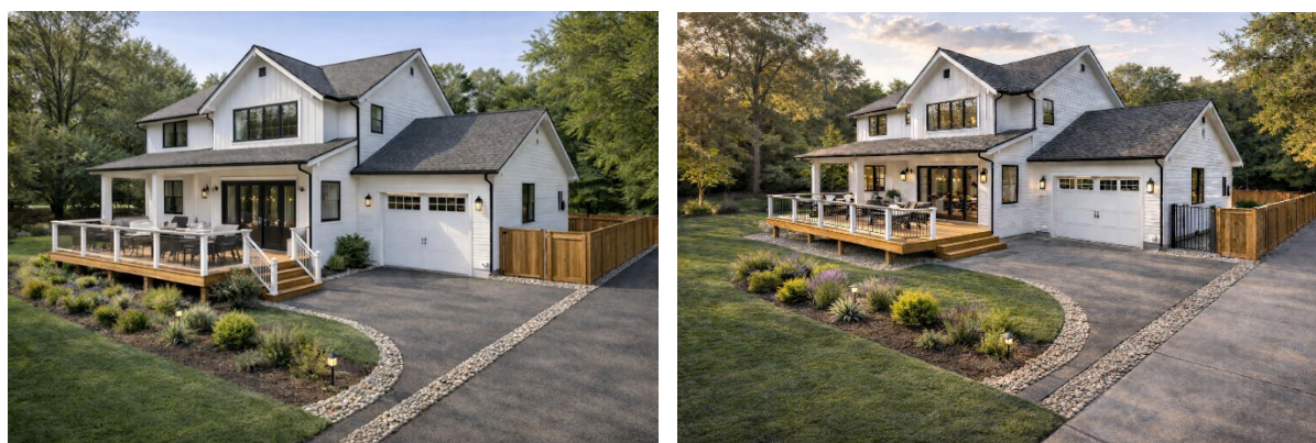
Figure 3. Before-and-after image of a single-family house that implemented Zone 0. Note the relocation of the plants away from the deck and the installation of a noncombustible gate (courtesy of ChatGPT). While not required by this regulation, best practice is to install metal mesh screening around the perimeter of the deck to minimize debris accumulation and ember entry into the under-deck area.
