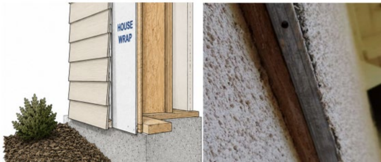
Figure 6. The image on the left shows a simplistic assembly of an exterior wall that illustrates sheathing, house wrap, and siding (courtesy of ChatGPT). On the right is a photo of the base of a stucco wall with the sheathing visible behind the weep screed (photo courtesy of Steve Quarles). Without proper flashing, the sheathing and house wrap can be vulnerable to flames and allow fire to enter the wall cavity.
