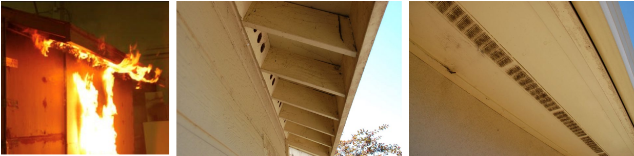
Figure 7: The left image shows flames trapped under the eave. The middle image illustrates exposed rafters and freeze-block venting in the blocking. The image on the right shows a soffited eave and strip vents. All images courtesy of Steve Quarles.
