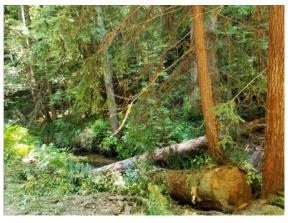
Crews use a log skidder to place large woody debris into Hare Creek. Note the location wedged between the redwood and tanoak on the bank to protect the log from moving downstream during high flows.
