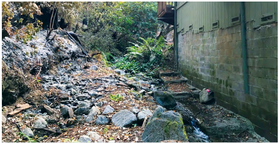
CZU Complex VAR 48. A house adjacent to Foreman Creek with high debris flow and flood hazards.
