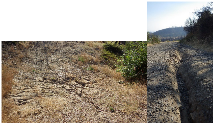
Figure 4. A road surface with rills (Left) and a gully formed (Right).
