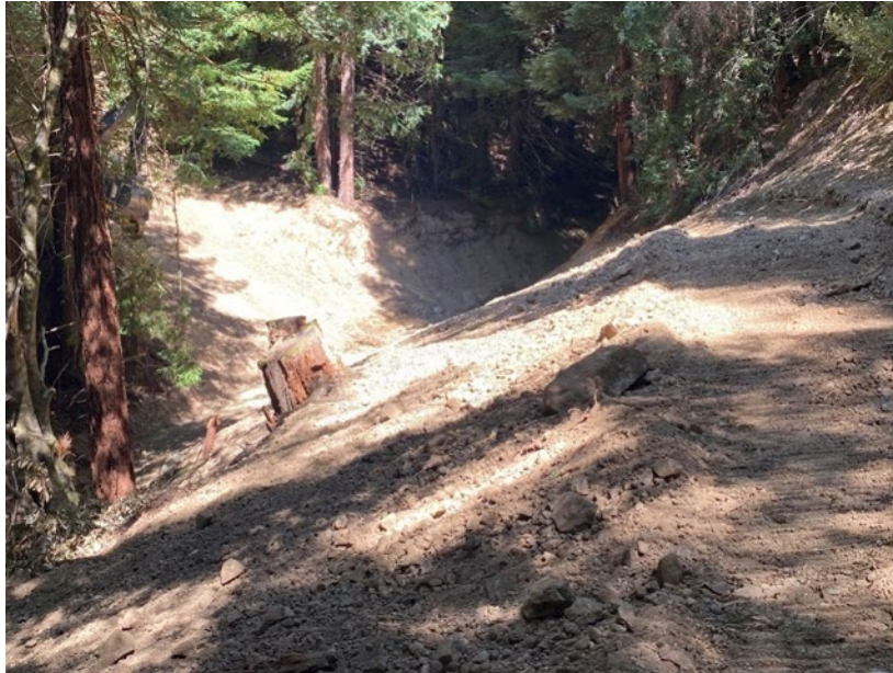
Large Class II In-Stream excavation, Road 110
