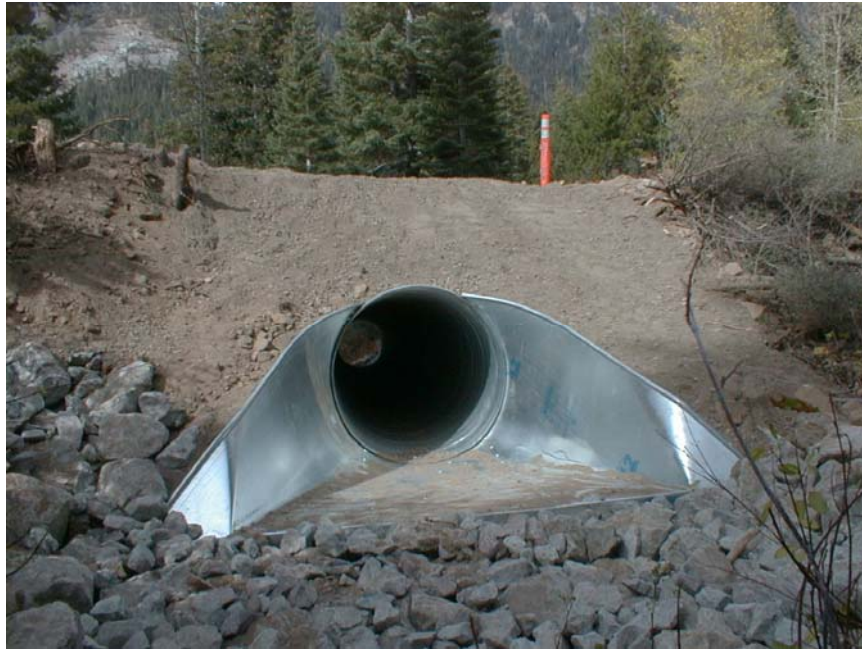
Figure 11. Example of a metal flared end section (photo provided by Mike Derrig, USFS).
