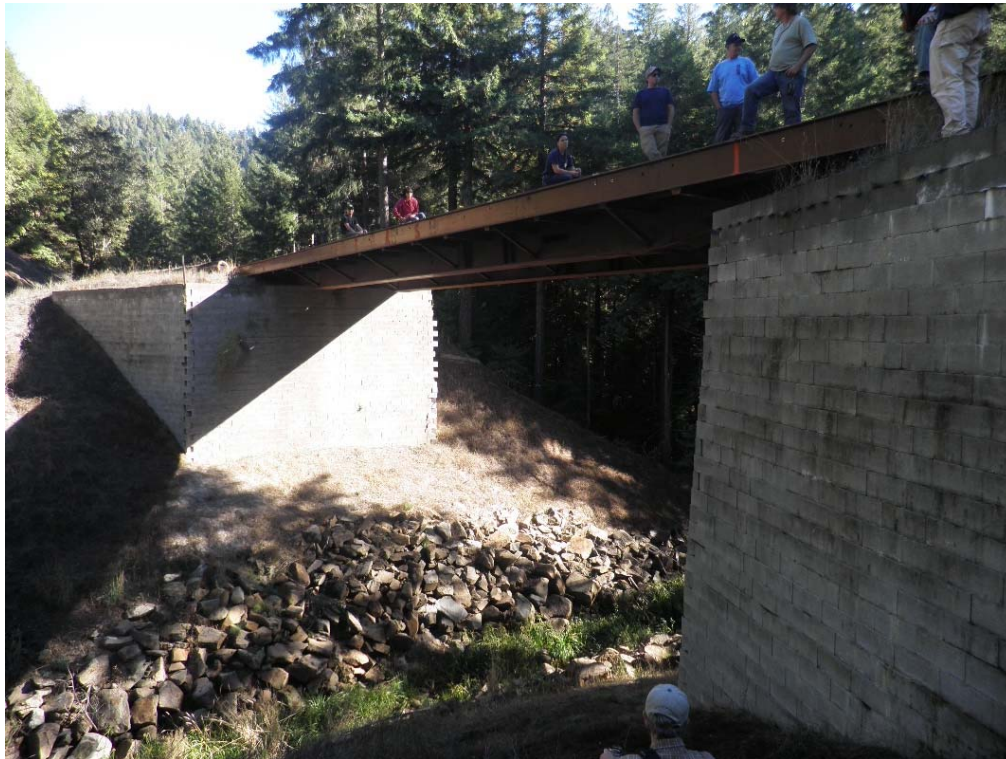
Figure 31. GRS bridge abutments founded above the Q_{100} water surface elevation, Mendocino County (photo provided by Gordon Keller, USFS (retired)).
