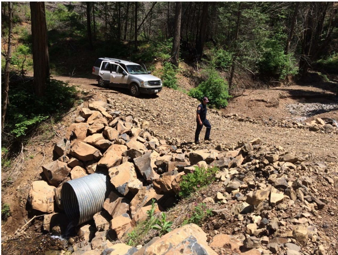
Figure 14. A vented rock-filled crossing that is subject to debris flows in northeastern California.
