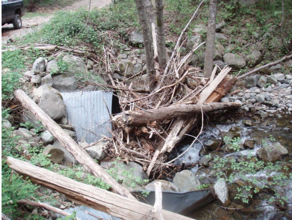
Figure 9. Woody debris blocking a culvert inlet in the upper Sacramento River watershed (photo provided by Matt Boone, CAL FIRE).
