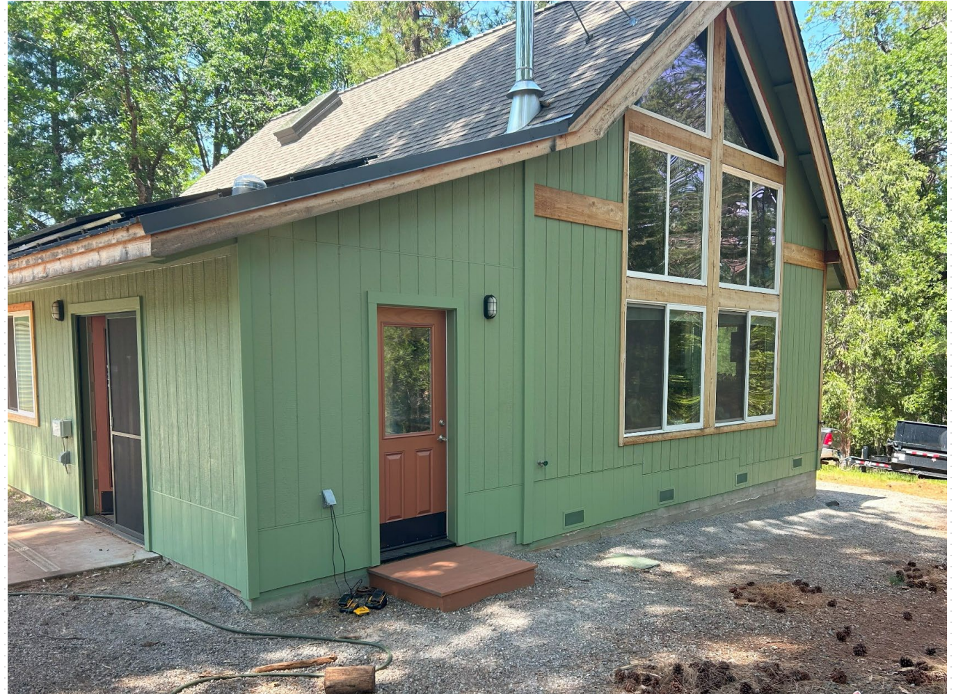
2' lower wall retrofit
