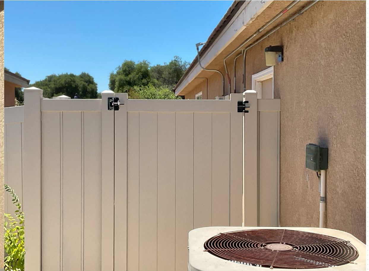
Replaced with Metal Gate and Fence
