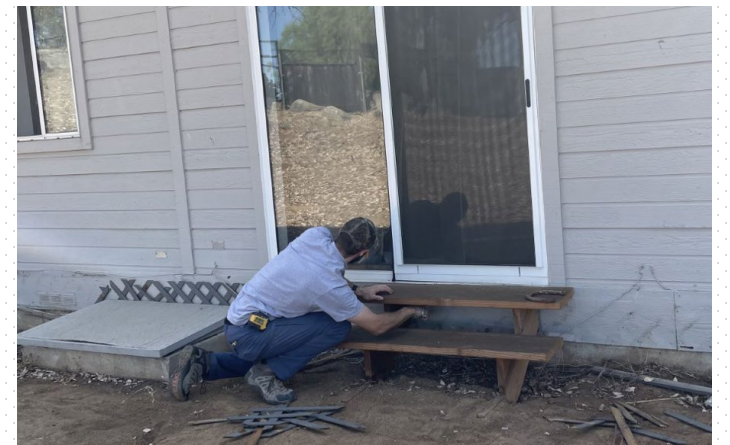
Removing the Combustible Skirting
