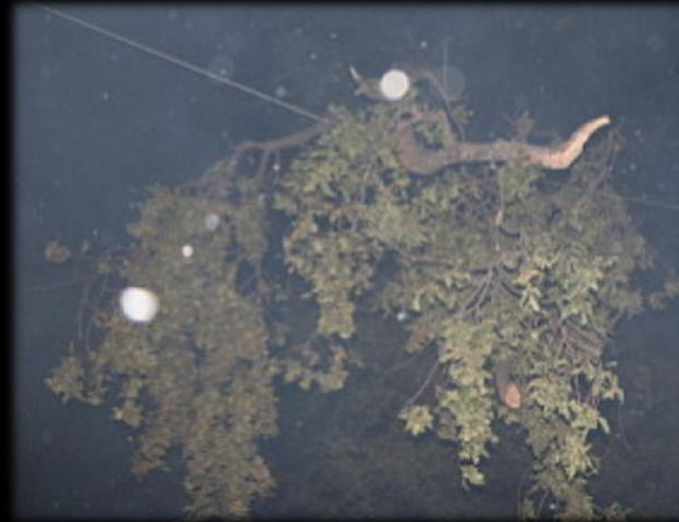
Branches across powerlines
