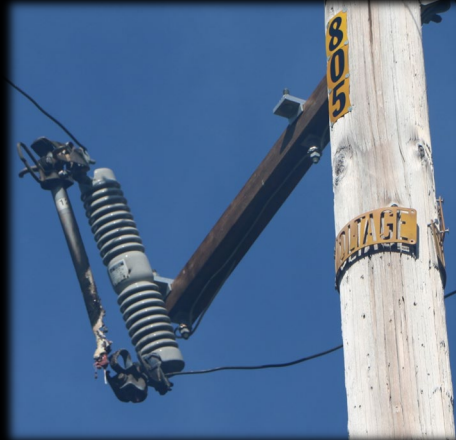
Fuse Failure
