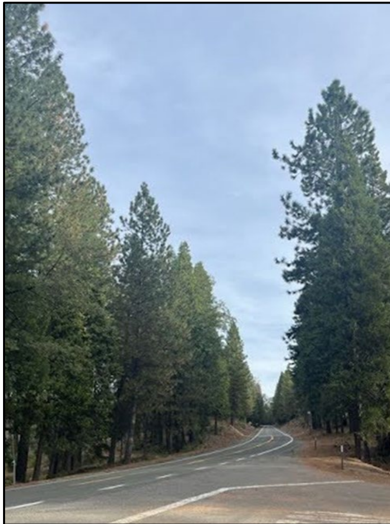
Figure 2.3. A typical road in a Butte County ridge community.
