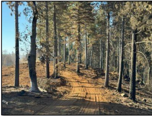
Figure 3 Images of treatment "HWY G Line HFR" showing decreased tree mortality within the treatment area. (date: August 8, 2024)
