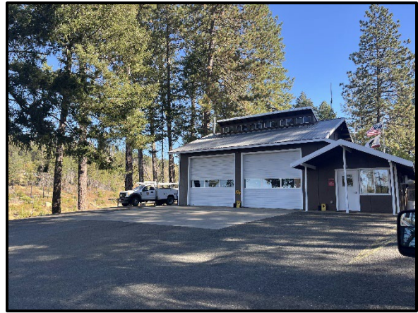
CAL FIRE Station 36 Jarbo Gap.
