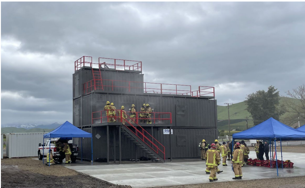
Figure 24 – TUU South Training facility at Porterville CAL FIRE Station
