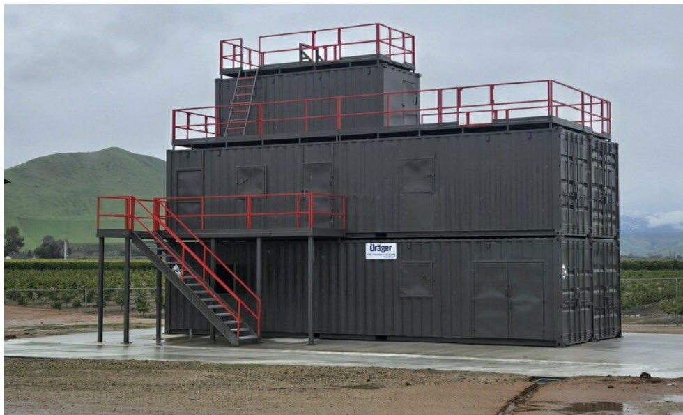
Figure 25 – TUU North Training facility at Woodlake CAL FIRE Station
