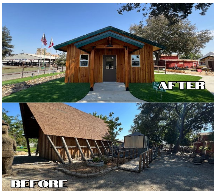
Figure 1 The renovated CAL FIRE booth at the Tulare County Fair.
