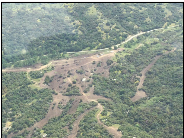
Figure 2 Crawford Corral project progress.
