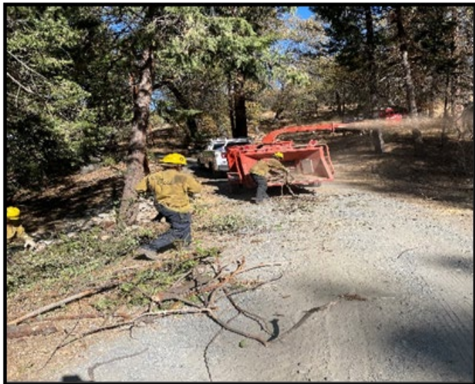
Figure 12 Crew clearing brush from roadway.
