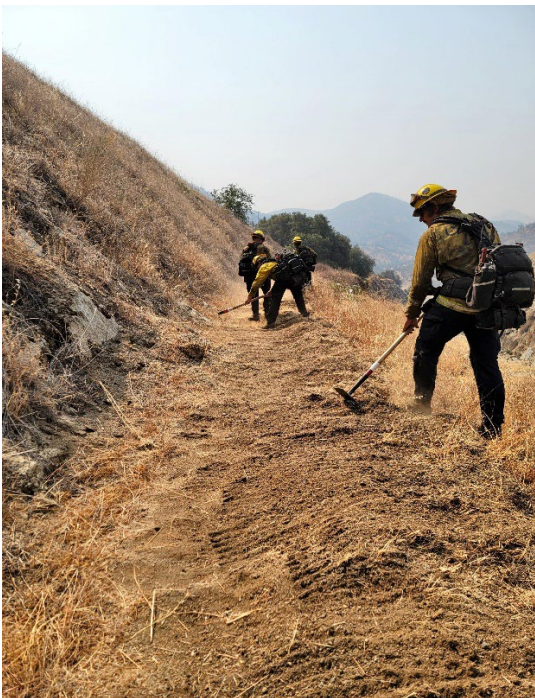
Figure 7 CAL FIRE hand crew constructing a fuel break.
