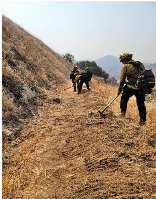
Figure 10 CAL FIRE hand crew constructing a fuel break.
