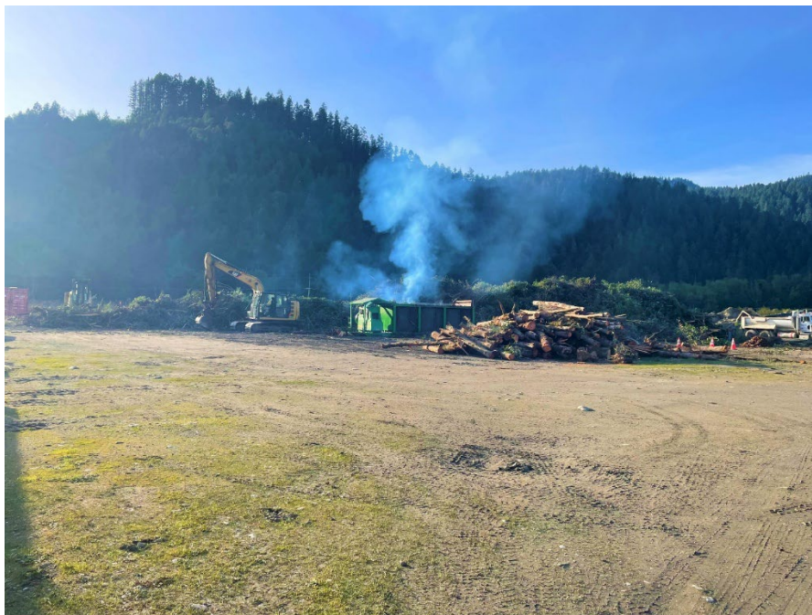
Image 7 Air Curtain Burner being utilized for storm damage clean-up in Willow Creek.
