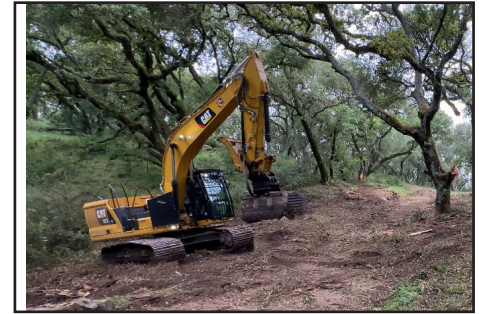
CAL FIRE excavator with masticator head
