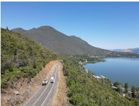
Roadside fuel reduction work along Soda Bay Road
