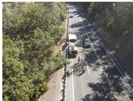
Roadside fuel reduction work on HWY 29 outside Lower Lake
