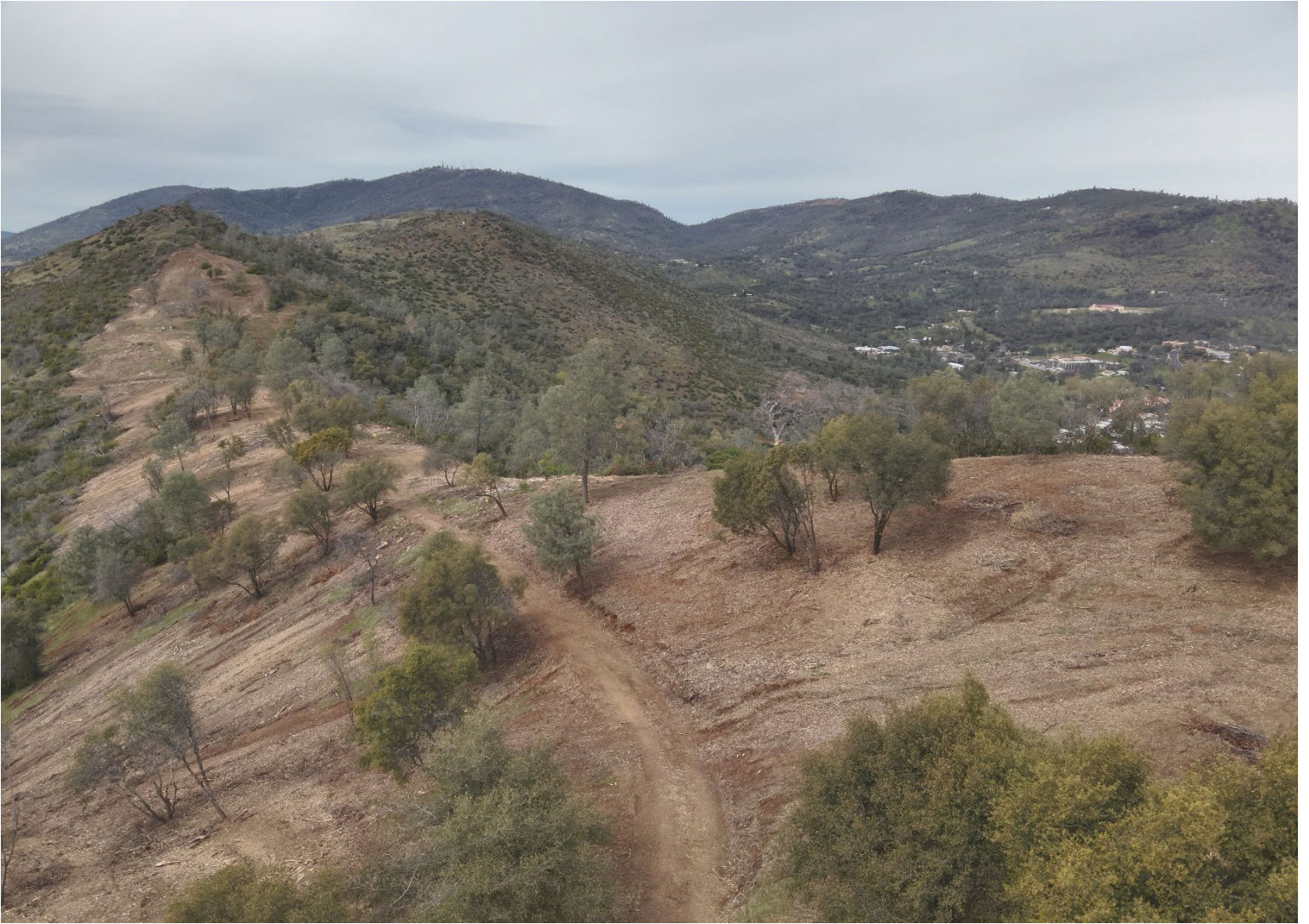
Bumgardner Shaded Fuel Break. Project completed by Mariposa Fire Safe Council.
