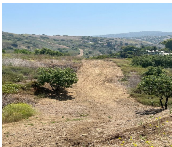
Olinda Village Fuel Break After Work
