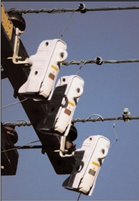
Figure NE-8: Enclosed Cutouts
