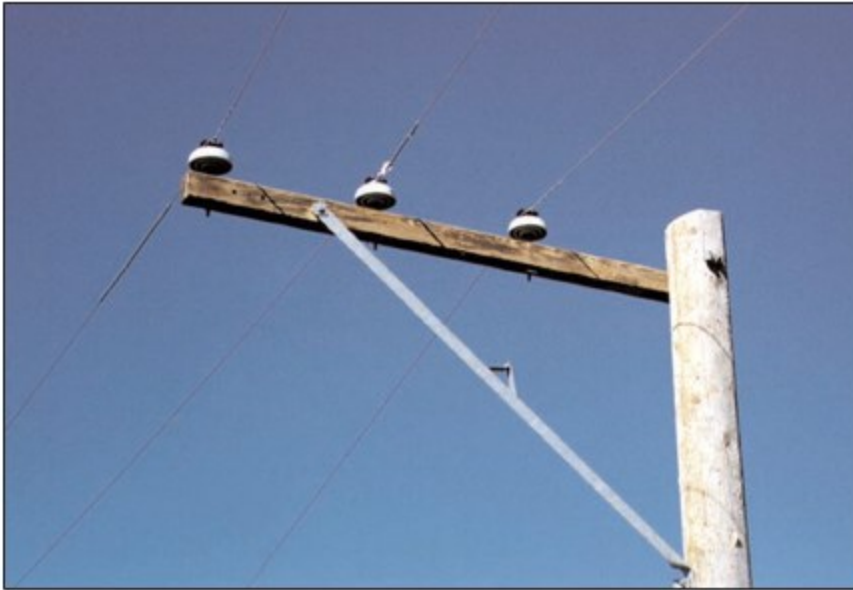
Figure PLC-3: Alley Arm
