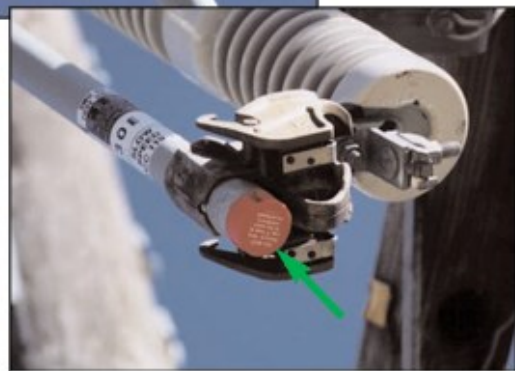
Figure B-17: SMU-20 - Fuse Detail
