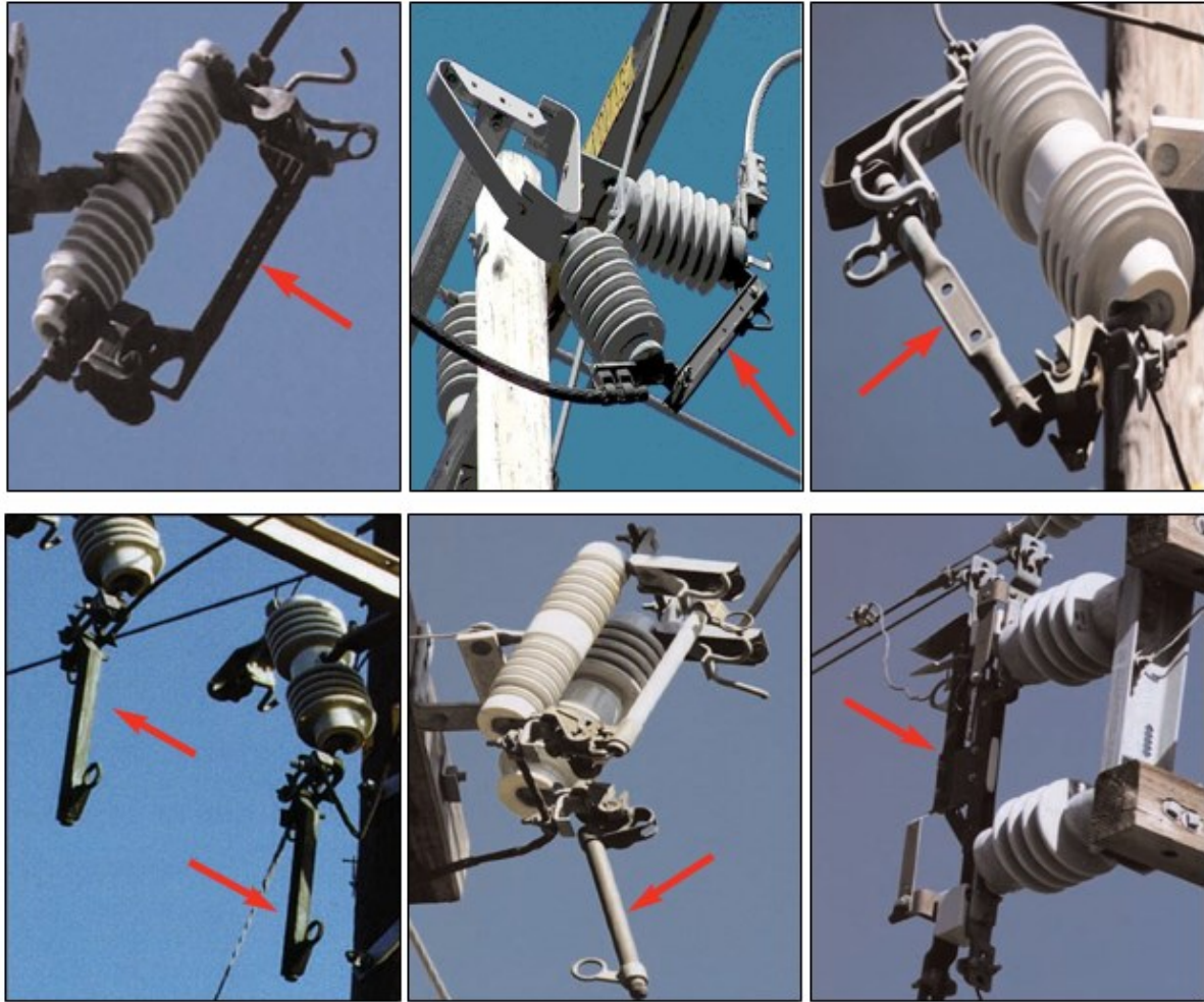
Figure NE-13: Solid Blade Disconnects
