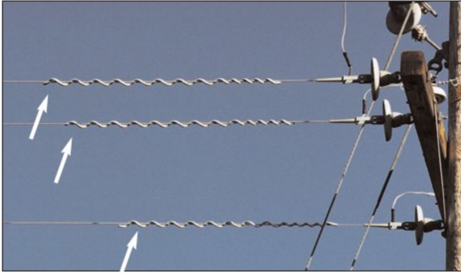
Figure PLC-13: Vibration Damper
