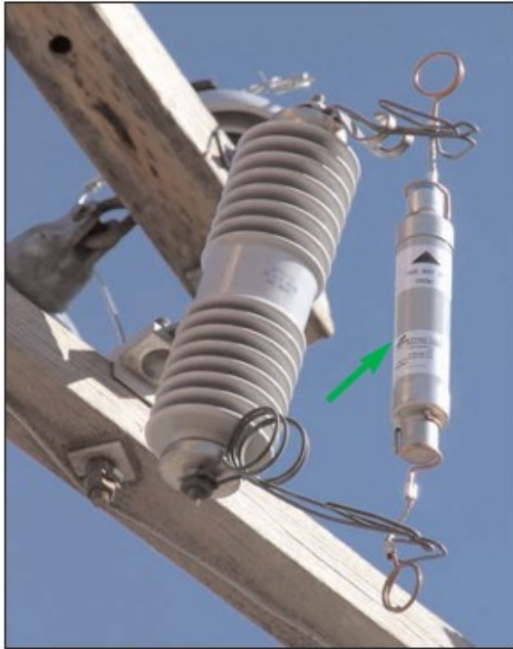
Figure B-12: Also Fits "Open Link" Cutouts
