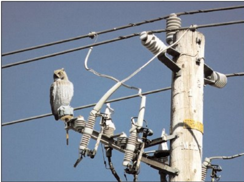
Figure PLC-20: Anti-Perch Owl
