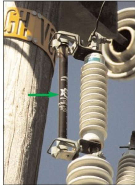
Figure B-11: Liquid Filled Fuse
