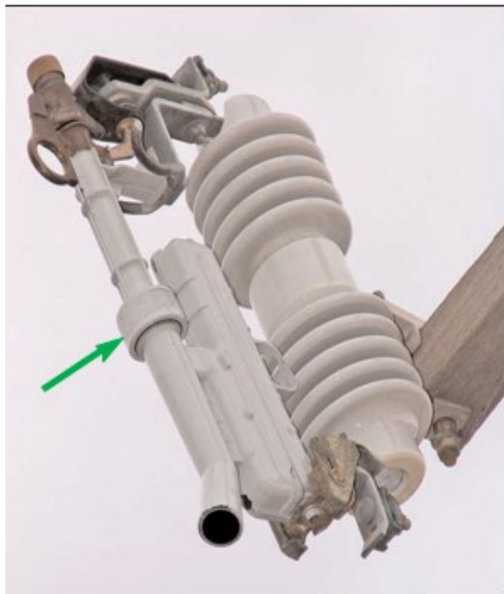
Figure B-20: S&C Fault Tamer Fuse
