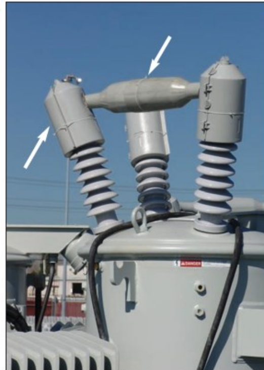
Figure PLC-26: Bushing Covers
