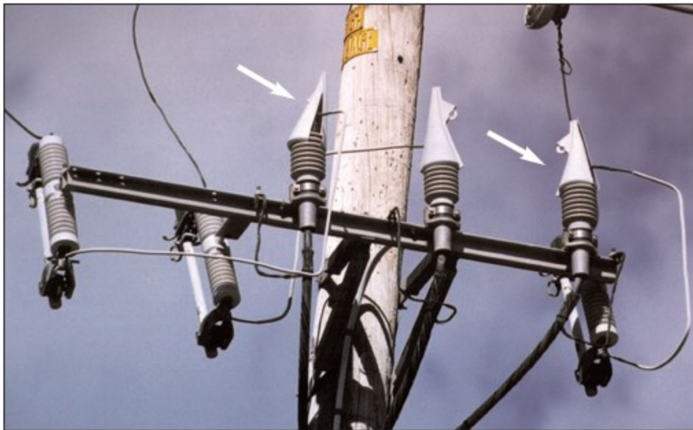
Figure PLC-22: Squirrel Guard
