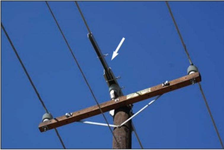
Figure PLC-24: Raptor Protection Insulator and Wire Cover
