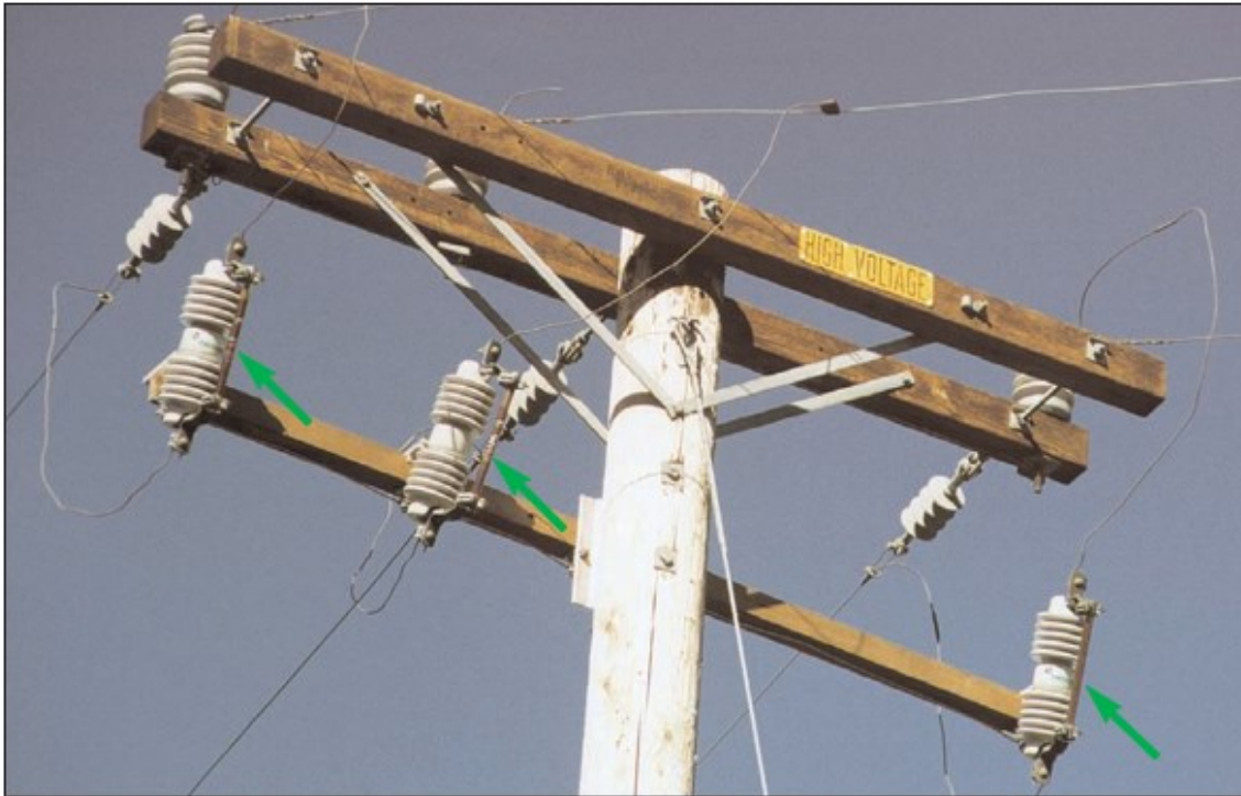
Figure B-8: Arm Mounted Cutout with Liquid Filled Fuse
