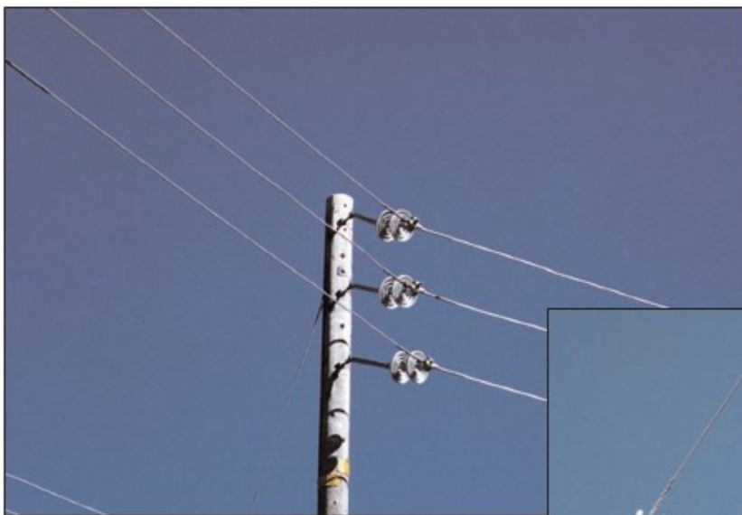
Figure PLC-1: Vertical Angle
