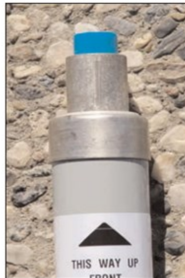
Figure B-15: Fault Indicator Cap Indicator Orange Band under Blue Cap
