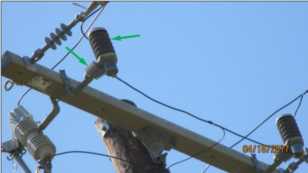
Figure B-86: Siemens Lightning Arrester
