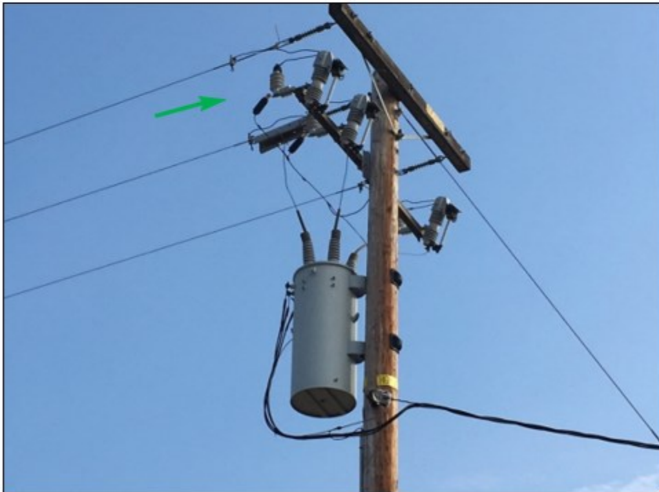
Figure B-88: ABB surge arrester equipped with Spark Prevention Unit (SPU), rated 10kA IEC Class I & II 44 kV and below
