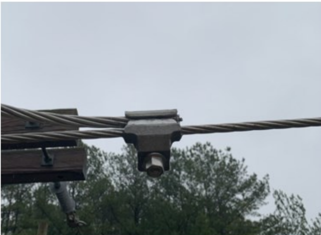
GA9000 Parallel Groove Connector on Conductor
