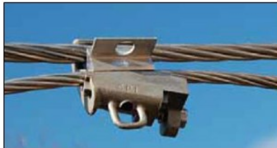
Figure B-71: CPI Wedge Connectors on Line
