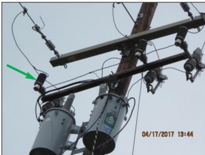
Figure B-87: Siemens Lightning Arrester
