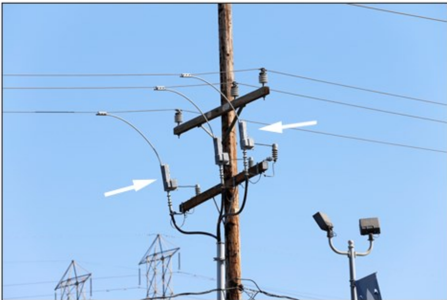
Figure PLC-15: Termination with animal protection cover
