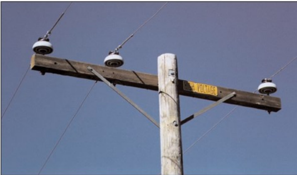
Figure PLC-4: Crossarm (Tangent)
