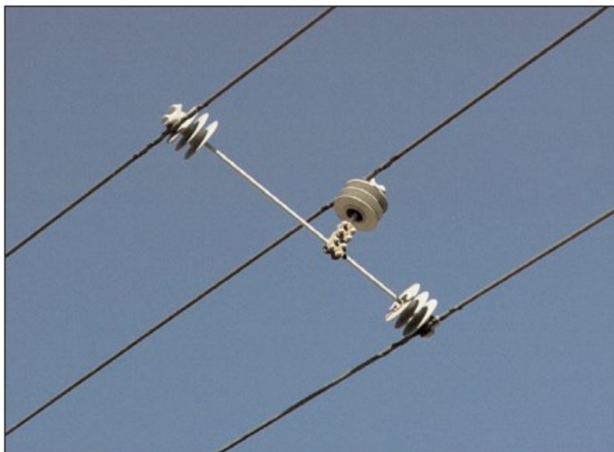
Figure PLC-12: Long Span Conductor Spreader
