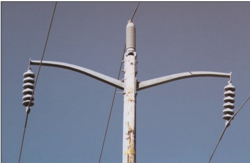
Figure PLC-31: Gull Wing
