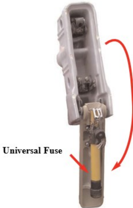
Figure NE-9: Open 4kV Cutout
