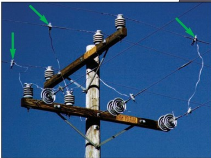
Figure B-60: Hot Tap Clamps on conductor
