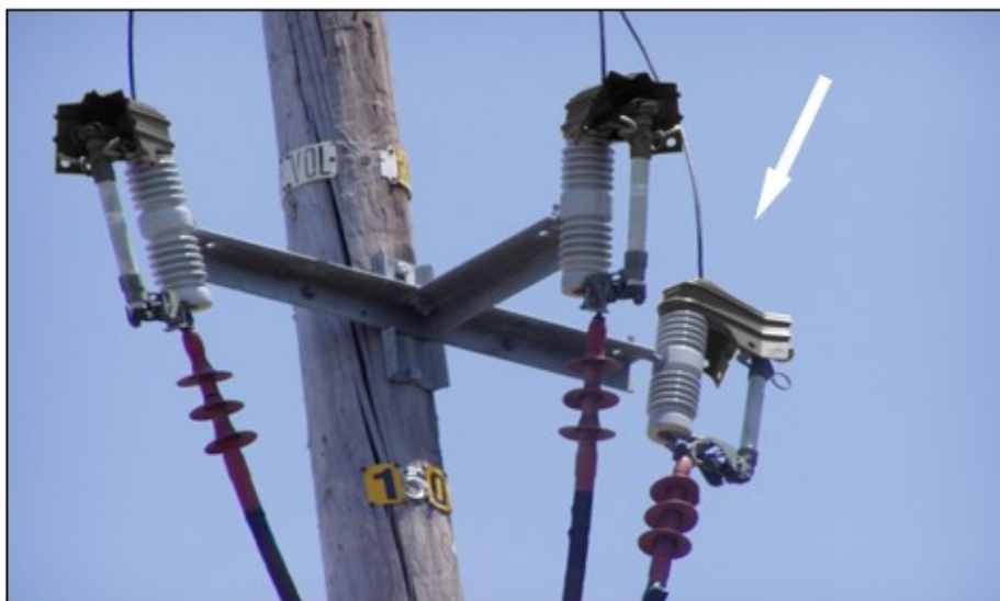
Figure PLC-16: Cut-out animal protection covers
