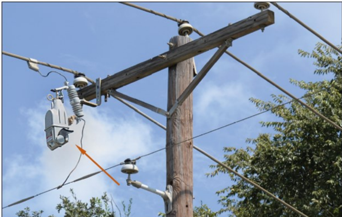
Figure A-7: Trip Saver II Cutout mounted single phase recloser with vacuum fault-interrupter
