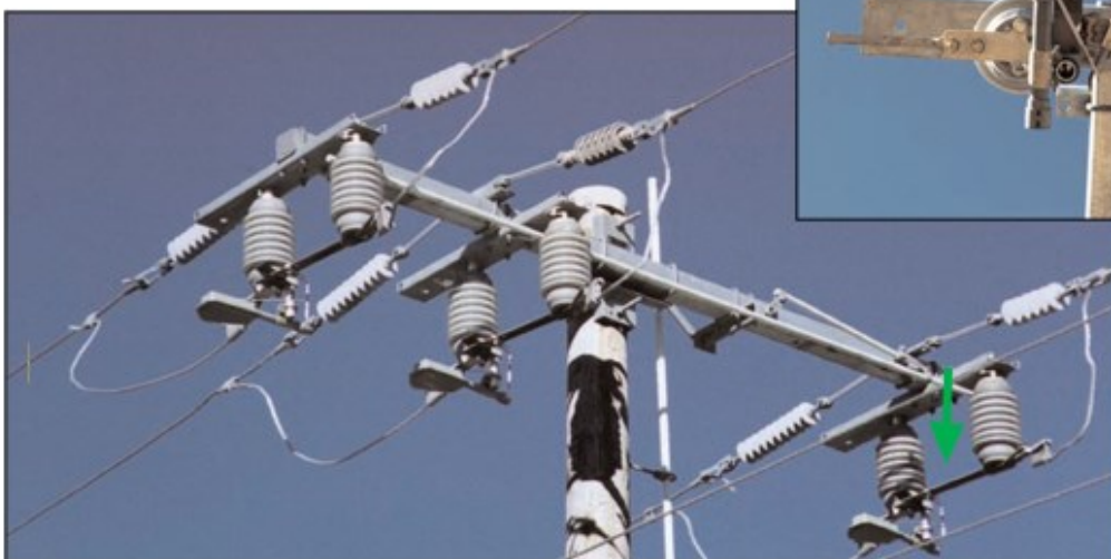
Figure B-29: Eaton-Cooper 600 Amp Underarm Side Break Switch (Closed Position)
