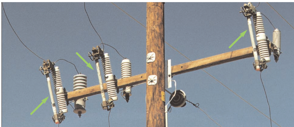
Figure 3-16 Arm Mounted Cutout with SMU-20 Fuses
