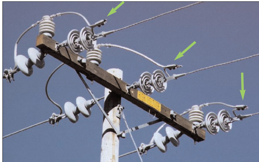
Figure3-48 Parallel Groove Connectors on Jumpers
