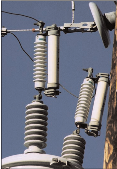
Figure 3-4 Bushing Mounted Cutout with Non-Expulsion Fuse
