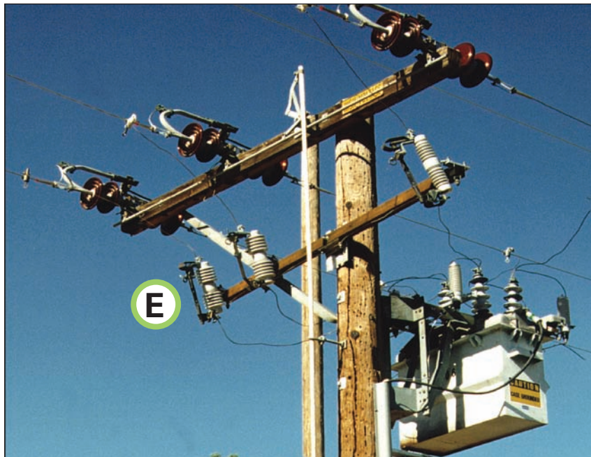
Figure 3-37 Recloser with Solid Blade Disconnects (closed position)
