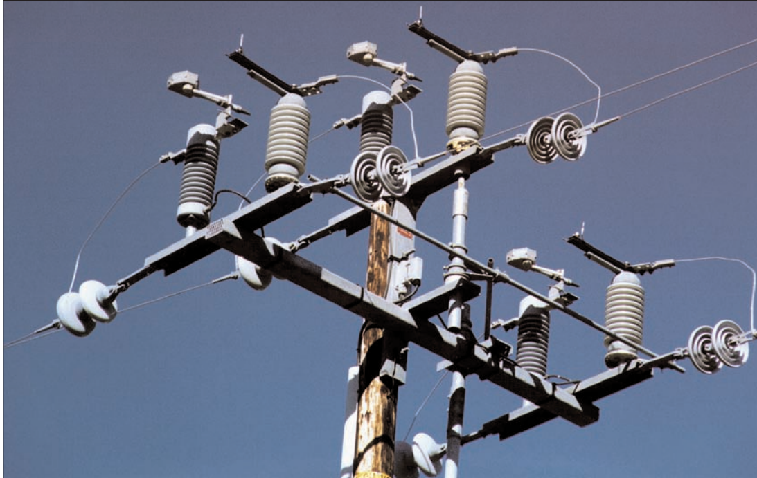
Figure 3-30 S&C Omni-Ruptor Switch, Triangular Construction (open position)
