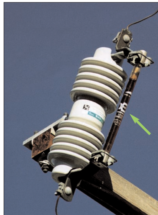
Figure 3-11 Liquid Filled Fuse
