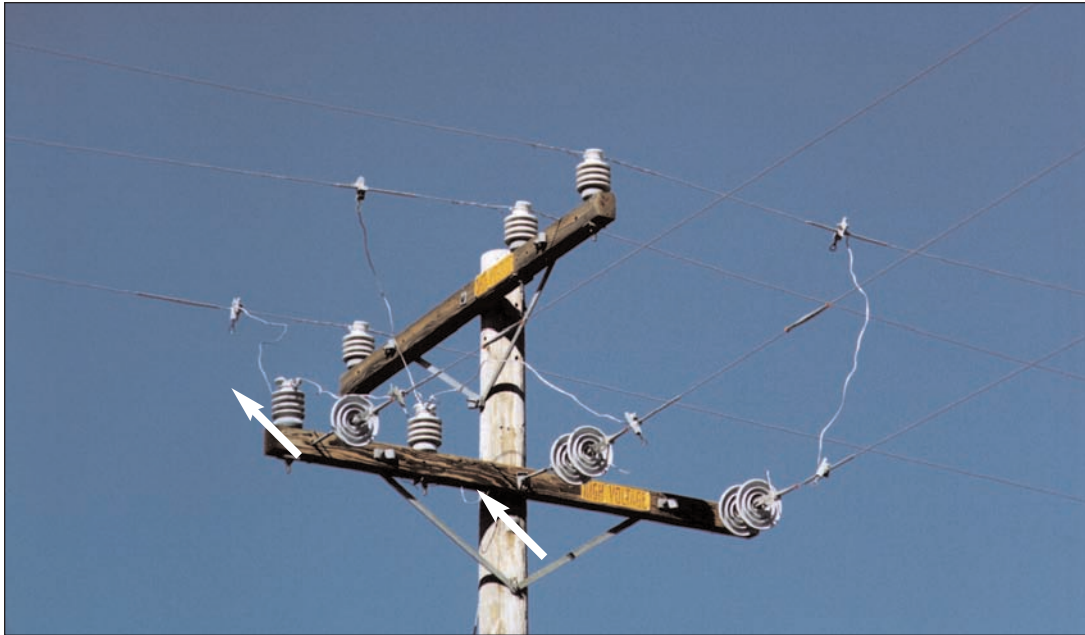
Figure 4-5 Tangent Crossarm with Deadend Tap (T-Tap)
