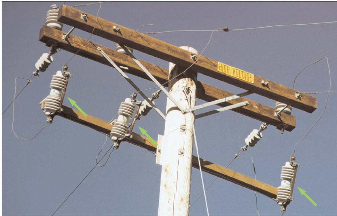
Figure 3-10 Arm Mounted Cutout with Liquid Filled Fuse
