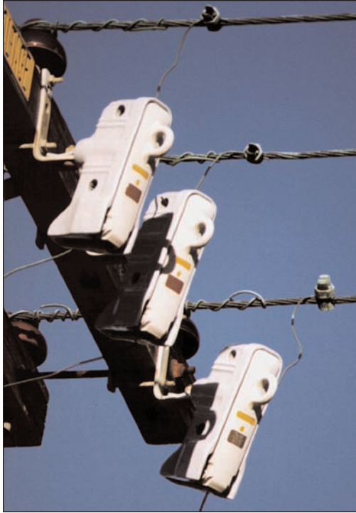
Figure 2-8 Enclosed Cutouts
