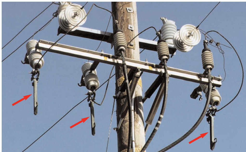
Figure 2-12 Arm Mounted Cutout with Solid Blade Disconnect (open position)
