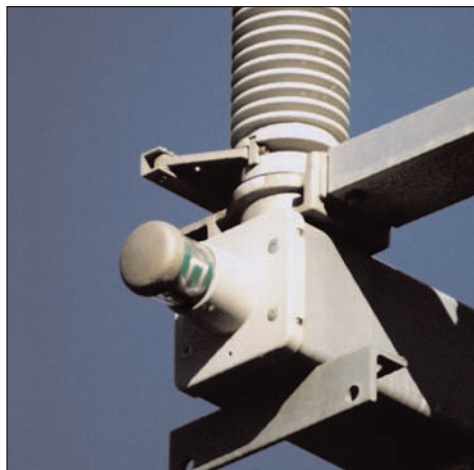
Figure 3-34 Open Position Indicator Green Letter "O" visible
