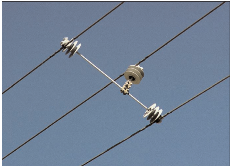
Figure 4-12 Long Span Conductor Spreader
