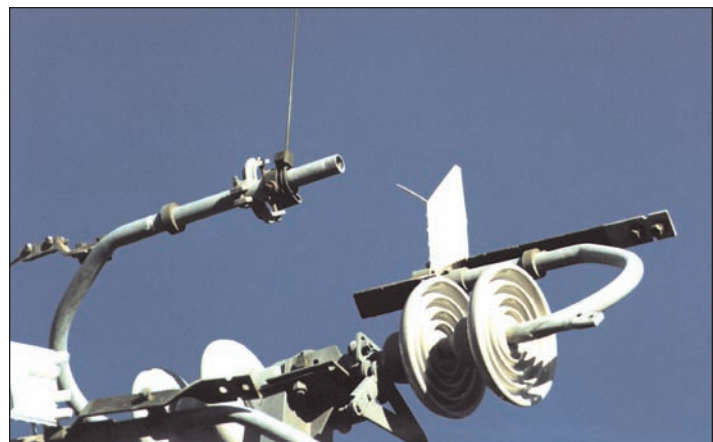
Figure 3-21 600 Amp KPF Air Switch, Triangular Construction (open position)
