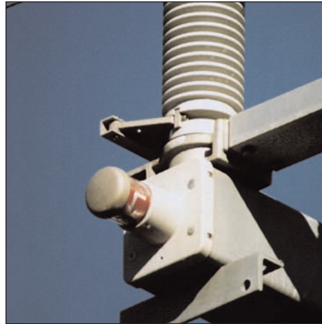
Figure 3-35 Closed Position Indicator Red
