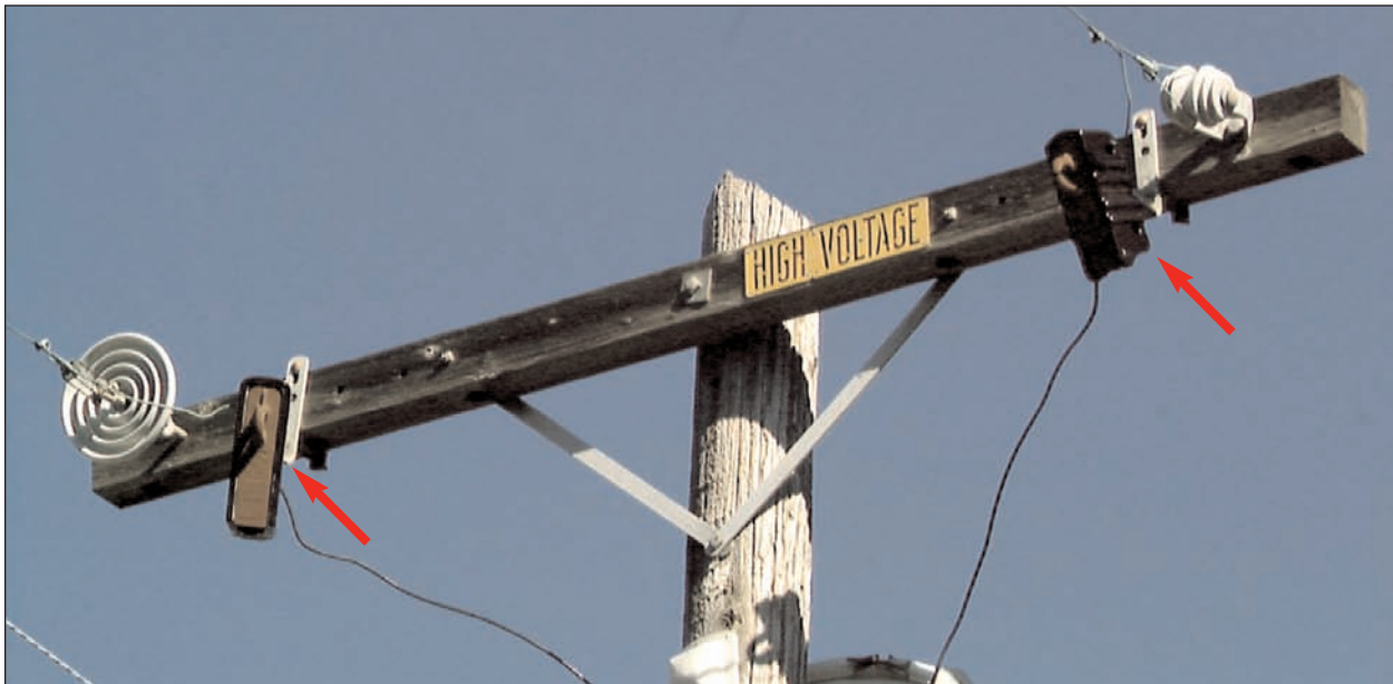
Figure 2-10 Arm Mounted Enclosed Cutout with Universal Fuses
