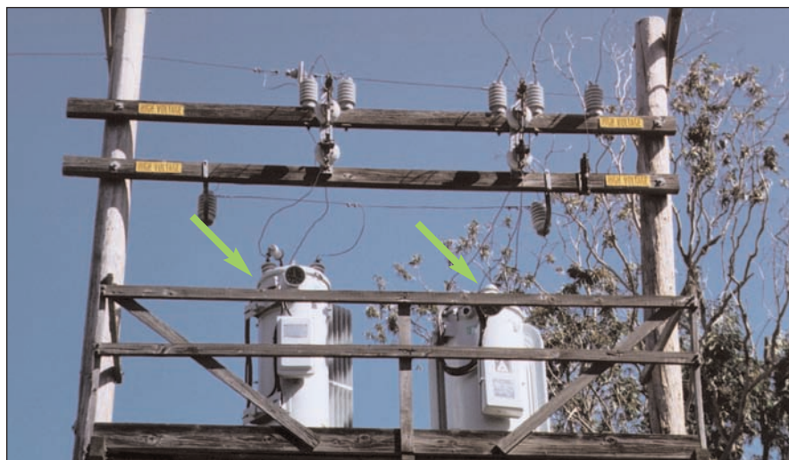
Figure 3-41 Voltage Regulator
