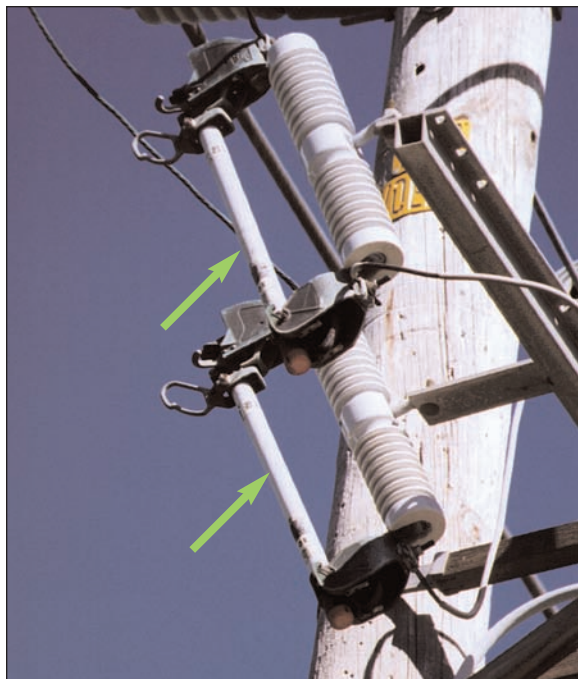
Figure 3-14 Arm Mounted Cutout with SMU-20 Fuses
