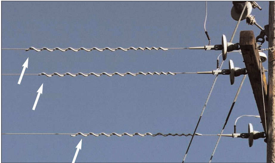
Figure 4-13 Vibration Damper
