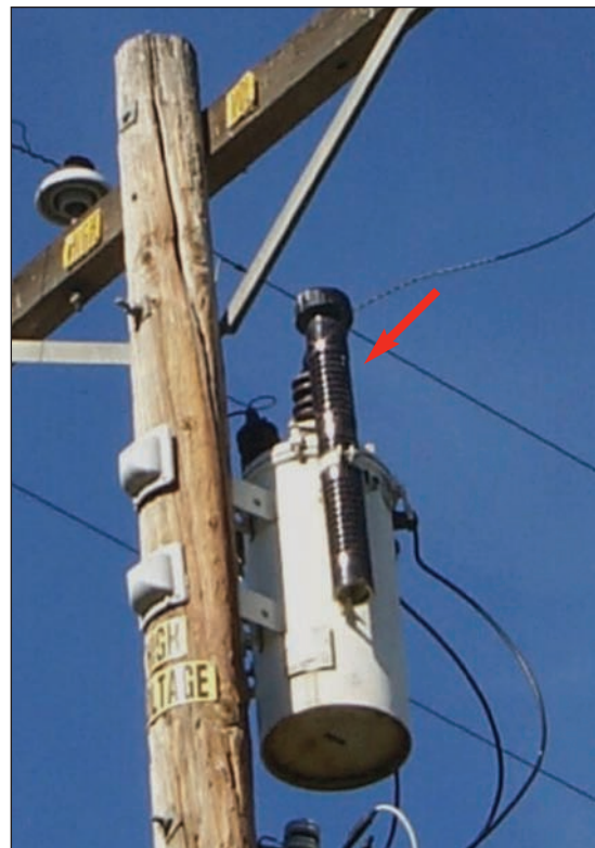
Figure 2-28 Lightning Arrester
