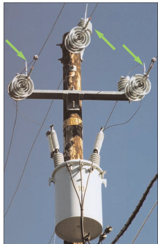
Figure 3-69 Automatic Deadends Attached to Pole and Crossarm
