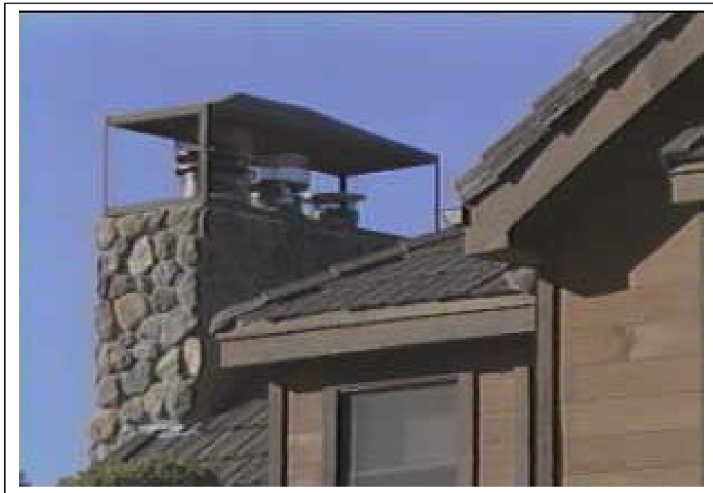
Photograph 11.2. Chimney/Stovepipes with Spark Arresters
