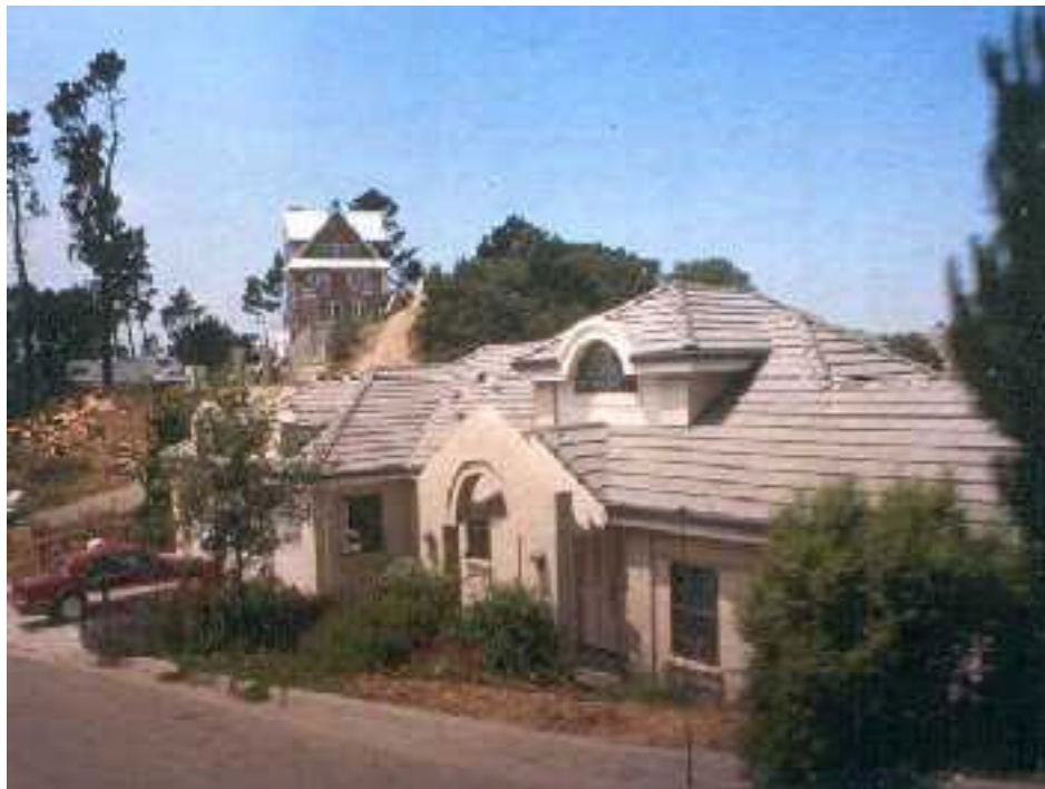
Photograph 11.1. A Clean, Well-Maintained Class A Roof
