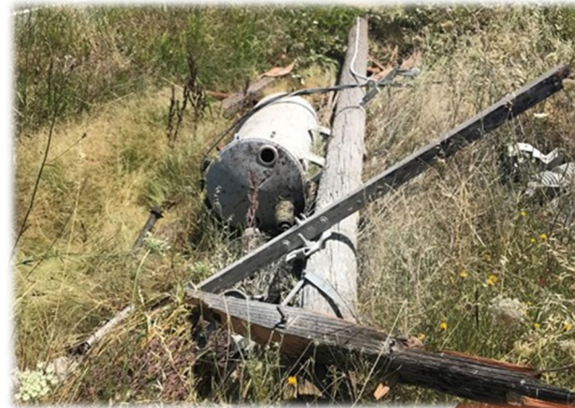
Vehicles contacting Power poles cause ignitions
