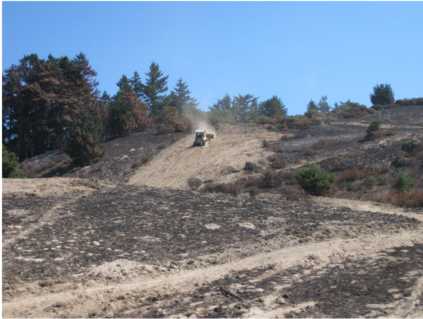
Post Fire Suppression Repair on the Lockheed Fire (2009).
